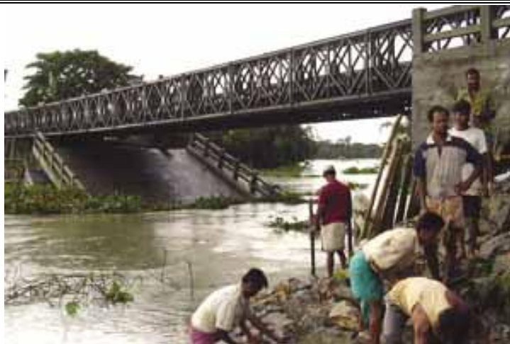
The Indian Army restored road communication by constructing a Bailey Bridge in NH 31 near Nalbari of Assam. The concrete bridge was damaged due to flood in 2004.
